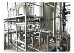
At the same time, we modernized the existing CIP station, replacing old sensors, instruments, valves and the control panel. A new regeneration water tank was added and the modernized CIP unit was integrated to the central automation and SCADA.
